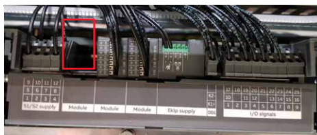
Fig. 4.3 Ekip Signalling or Com -module is possible to add to the Connection module of the draw-out switch powered by the auxiliary power supply module = Ekip Supply module
